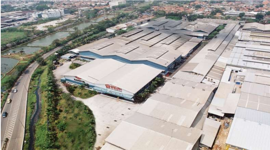
Kapuk Plant (Radiator Facilities)
